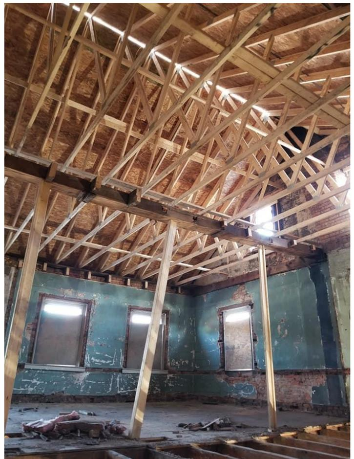
Freshly installed OSB-sheathed trusses form the roof’s new skeleton above the second floor, where flames had shot through some 17 months before, in a space historically used as residential living quarters. Photos dated 31 Dec. 2020.
