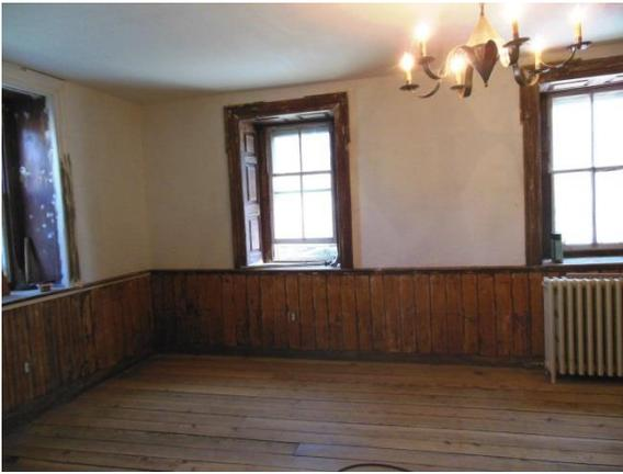
Floor sanding in progress, with now invisible window trim repair - custom-milled to match a missing corner.
