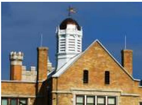
The restored parapet, the wall at the front entrance extending well above the roof line and flanked by two great towers, features a new clock face and restored decorative terra cotta embellishments. The striking metal dome of the large cupola/bell tower, which rises above the parapet and can be seen from many blocks away, is an Annville landmark. The replacement windows are now not only energy efficient, but they are historically correct.
